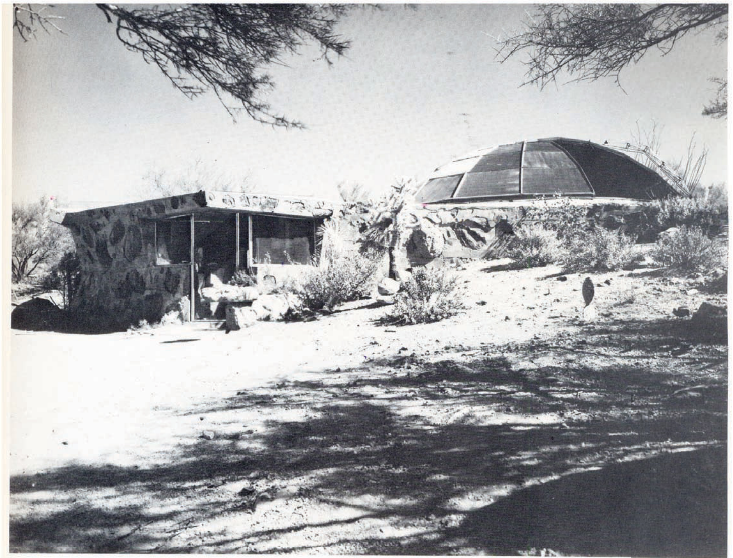
The entry, with the dome beyond. (© 1985 Julius Shulman)
